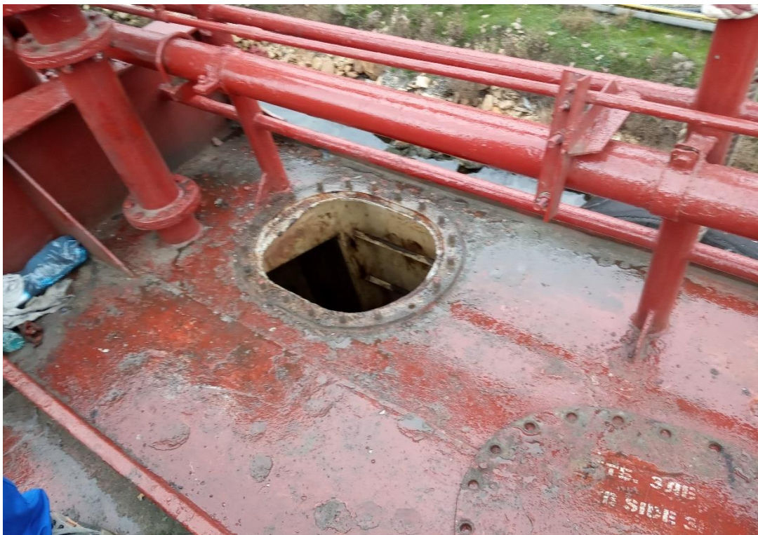
Fig.2. Manhole of ballast tank No. 3 – port side
