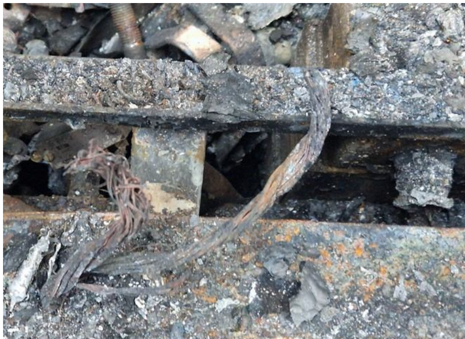
Fig. 4.11. Image of the feeding cables of the engine compressor
