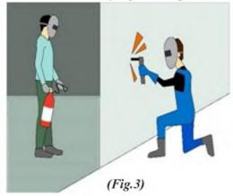
as well as in instruction WI-02-003/2013. The presence of fire surveillance in the adjacent premises during hot works(Fig.3) would give a possibility to prevent such incidents.
