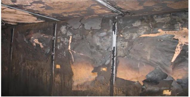
Fig. 15 Damages caused by fire in room № 2
