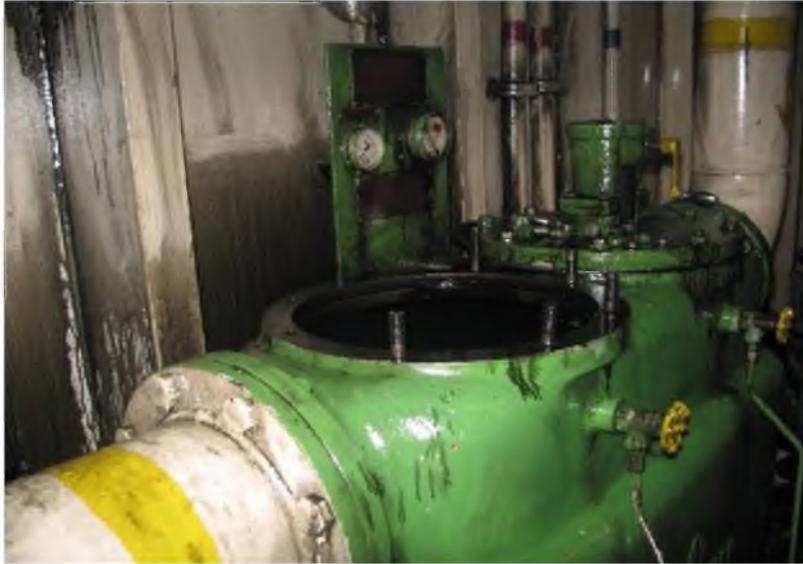
The eight nuts securing the cover of the section were unscrewed and put apart, but the cover was not detached from the housing - due to the sticking of its gasket and the fact, that part of the studs were distorted (**Fig. 8**). This made it difficult for the cover to move freely and even with the nuts unscrewed, it was likely that it to be held in place by the studs. The several attempts to remove the cover were unsuccessful.
