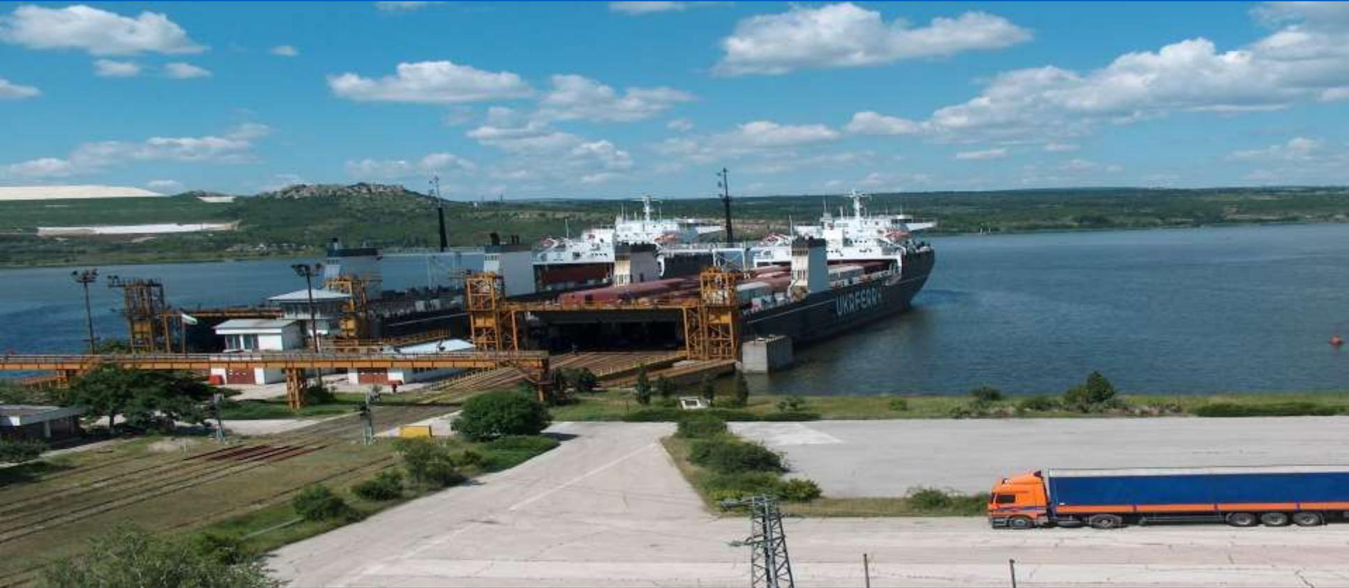
**The Ferryboat Terminal Varna has two berths, equipped with bridge gantries with five 1520 mm railway tracks each. The ferryboat terminal has the capacity to handle a ferryboat carrying 108 railway cars for 10 hours, and a ferryboat carrying 45 railway cars for 2 hours. The berths can accommodate two ferryboat vessels, 26 m and 22 m wide, respectively.**
